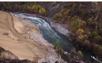
This is the beginning of the largest dam removal and river restoration project in U.S. history. As you can see with the removal of Copco 2, a free-flowing river is beautiful. By October, 2024, the remaining three dams will be out of the river, providing access to more than 400 miles of the upper Klamath watershed to spawning and rearing salmon and steelhead.
