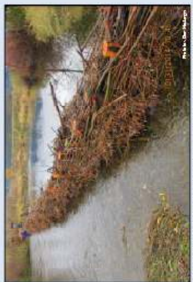
Example of willow weave construction at a Scott River PAWS site
